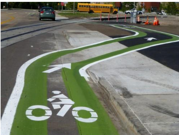
Figure 11. Example of a bike lane that is angled to guide bicyclists to cross railroad tracks safely. Source: Adam Farabaugh, ILoveBicycling.com
