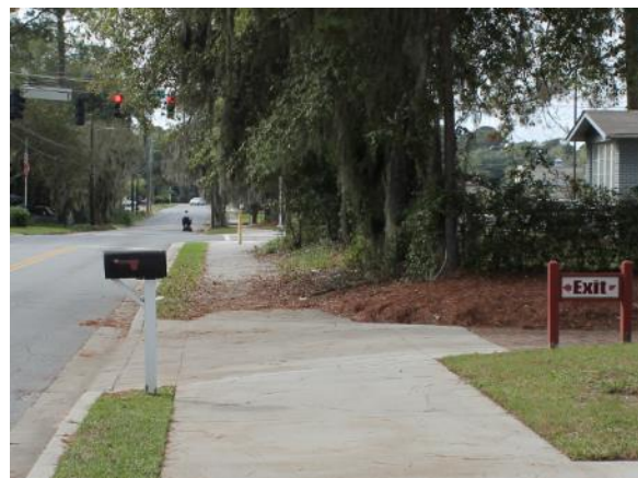
Figure 18. Accumulation of debris on a shared-use path in Valdosta, GA. (Photo: Ariel Godwin)
