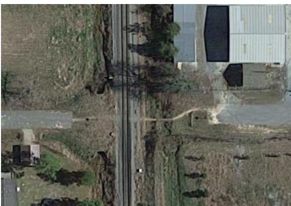
Figure 13. Aerial view of a “cow path” across the railroad tracks on Sheridan Street. Source: Google Maps.
