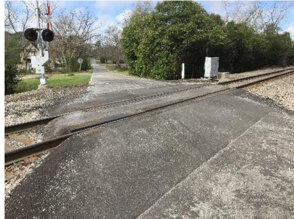
Figure 9. Angled railroad crossing on West Oconee Street.
