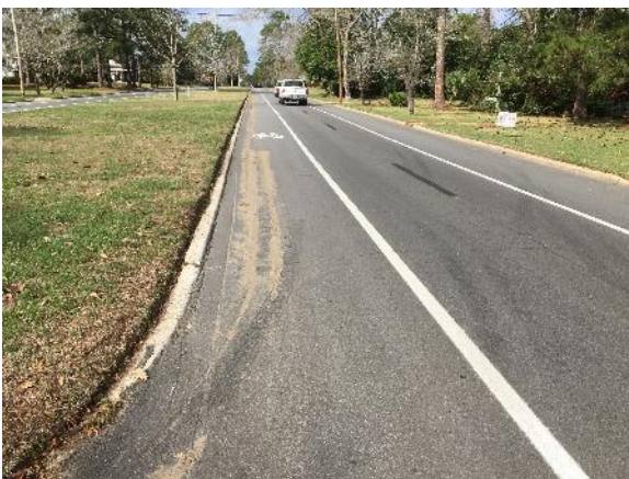
Figure 17. Accumulation of debris in the Central Avenue bike lane in Fitzgerald. (Photo: Ariel Godwin)
