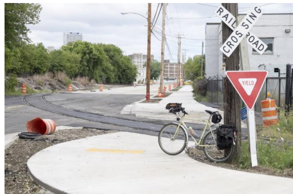
Figure 12. Example of a shared-use path that is angled to guide bicyclists to cross railroad tracks safely (Milwaukee, WI). Source: Dave Schlabowske, Urban Milwaukee.
