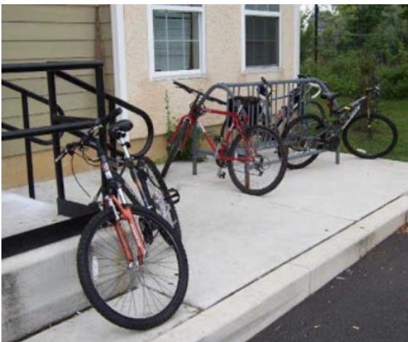
Figure 1. Older style of bicycle rack, colloquially known among cyclists as a “wheel bender.” Note how bikes have been locked to the ends of the rack to avoid the wheel-bending effect, and one cyclist has avoided using the rack altogether. Source: First State Bikes ( http://www.1stbikes.org/2013/05/youtube-video-ban-wheelbender-bike-rack.html ).
