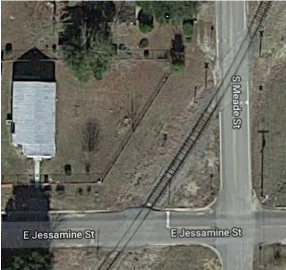
Figure 8. Angled railroad crossings near the intersection of South Meade Street and East Jessamine Street. (Source: Google Maps)
